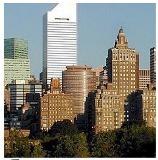
The designer met code compliance for wind loads and in so doing missed the critical load case - high windlass on the corners and not the face of the building.
