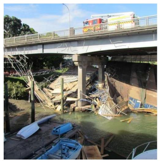
In 2017, the scaffold collapsed while seven workers were completing maintenance work on the bridge in Panmure. Six workers fell into the water and another was trapped on the scaffolding. No-one was seriously injured.
